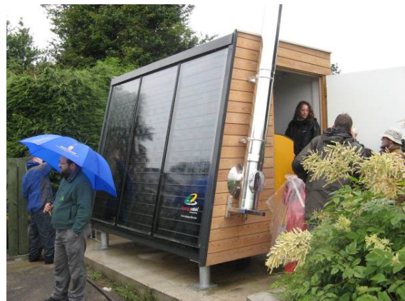
Figure 9. The Energy Cabin for supply of domestic hot water (solar) and biomass heating (Photo: P. Burgess).
