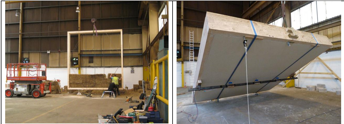
Fig. 19. ModCell® large wall elements - finishing: 30 mm external render & internal plaster
