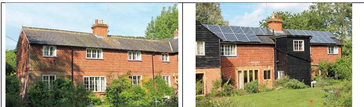
Fig. 21. The author’s cottage in Kent with timber stud wall upper elevation and rear extension
